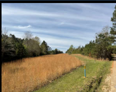
View of Pipeline from Rd
