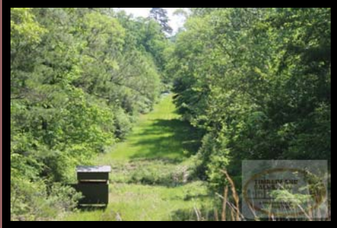
View along Pipeline
